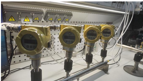
Fig. 5 Installation of transducers
